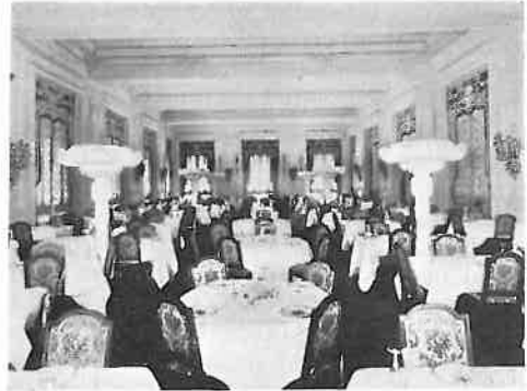
"Eye-Rest" lighting with pedestal fittings in hotel dining-room. The Mazda lamps and X-ray reflectors are fitted into the bowls of the pedestals.
