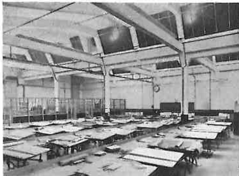
The lighting of this drawing office is carried out in an interesting and very effective fashion. Upturned silvered-glass trough reflectors containing Mazda lamps are fixed along the top of the concrete beams, and the light is thrown on to the long slope of the saw tooth roof, whence it is uniformly diffused over the working plane.
