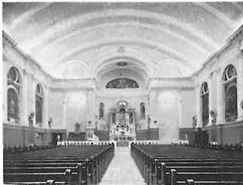
In this Church cornice "Eye-Rest" lighting is employed, the Mazda lamps and X-ray reflectors being concealed in a recess behind the cornice.
