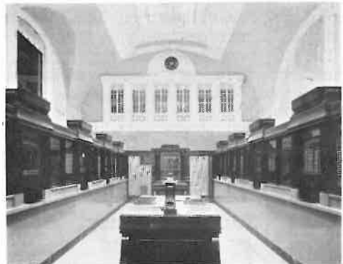
Bank lighting by means of X-ray reflectors and Mazda lamps contained in the eight boxes or troughs on top of the partitions.
